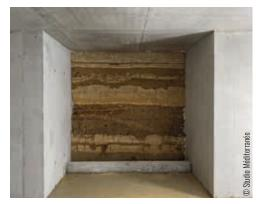
"This is a unique building project with a very low carbon footprint. Very few lorries came in and out of the building site. 80% of the materials were sourced on site, from the crushed concrete from the old winery and soil excavated by digging a gigantic 50-metre long and 12-metre deep hole. It's what you call cast earth or soil cement which involves casting soil as you would cement concrete".
